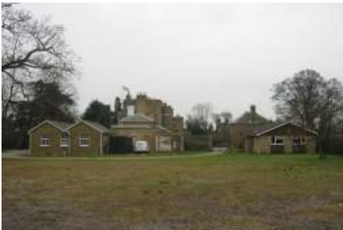
Fig 3.57: Stables and bungalow looking south towards Myddelton House beyond, 2003
