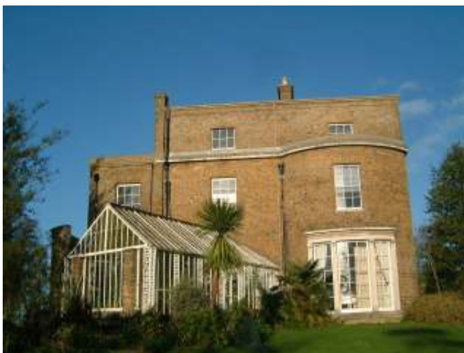
Fig 3.20: Myddelton House south elevation and angled conservatory, 2003
