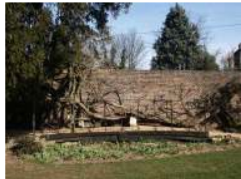
Fig 4.8: The listed Wysteria Bridge[17] over the New River, 2003
