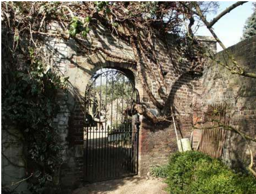
Fig 4.5: Kitchen garden/boundary wall, 2003
