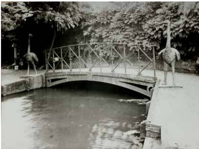
Fig 3.28: Wisteria bridge over the New River, c1920 (Myddelton House Archive)
