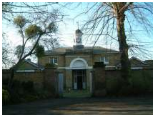
Fig 3.24: Stable yard entrance and front elevation, 2003
